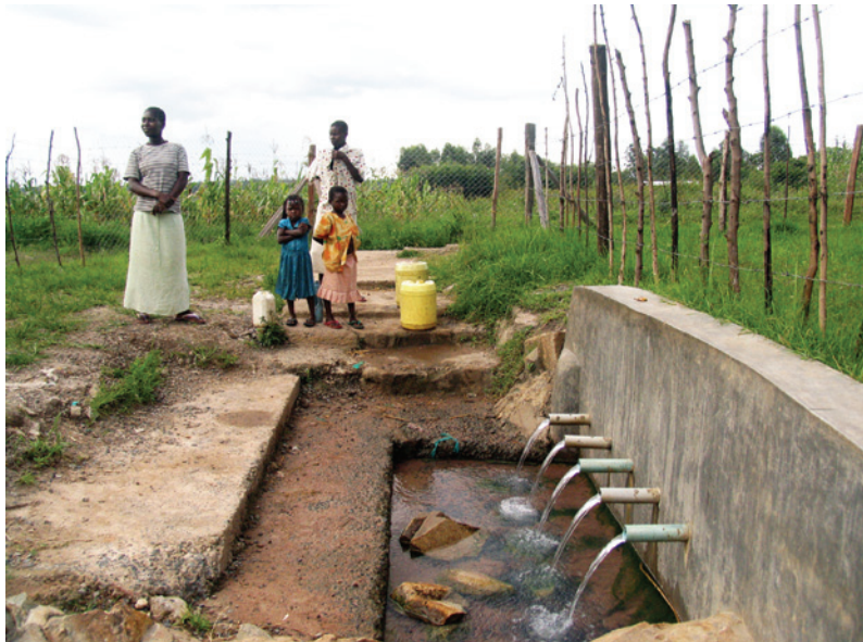
A rehabilitated and protected spring.
