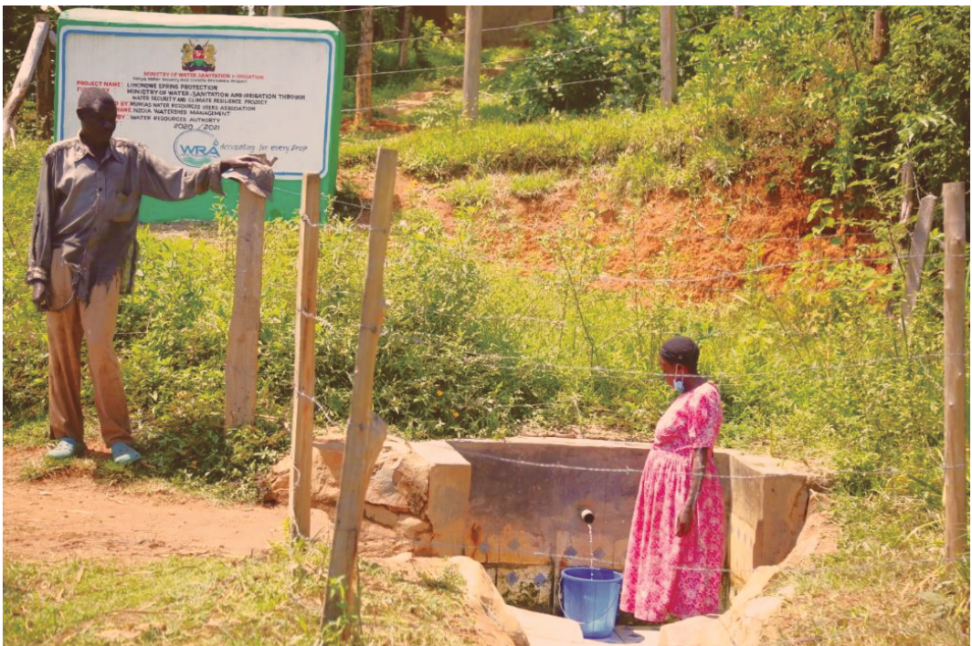
Fig.8. Spring protection done by Mumias WRUA in Nzoia watershed, Kakamega County, Lake Victoria North Basin
