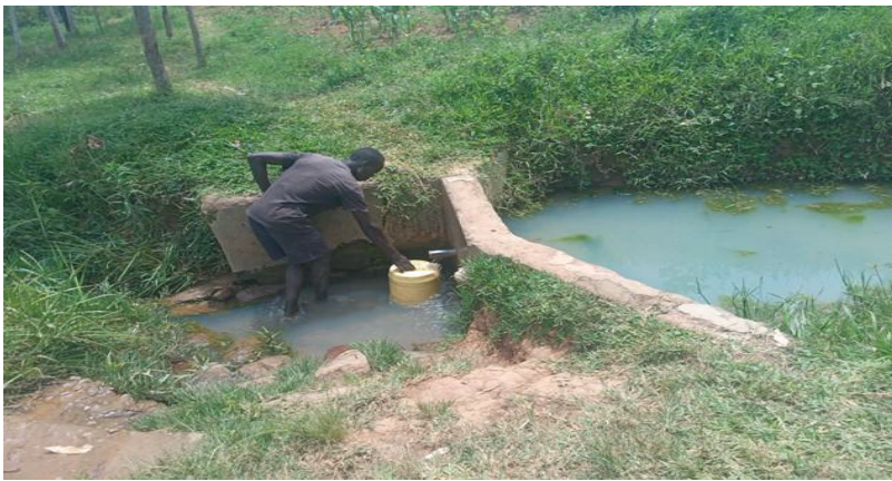
Fig.14. Unsatisfactorily managed protected spring
