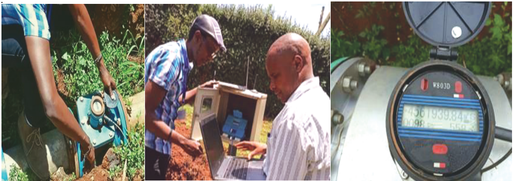
Fig.2. Installation of smart Meters
