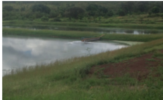
Properly implemented WDCP guarantees clean and safe water being discharged to the receiving water body
