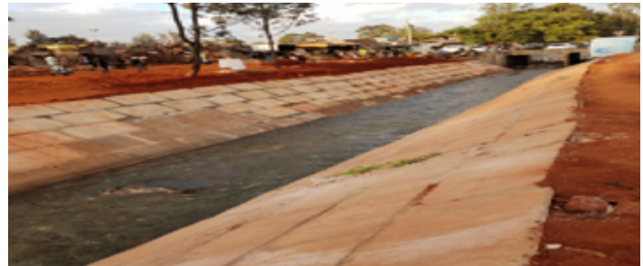
The degraded river bank and riparian land after rehabilitation
