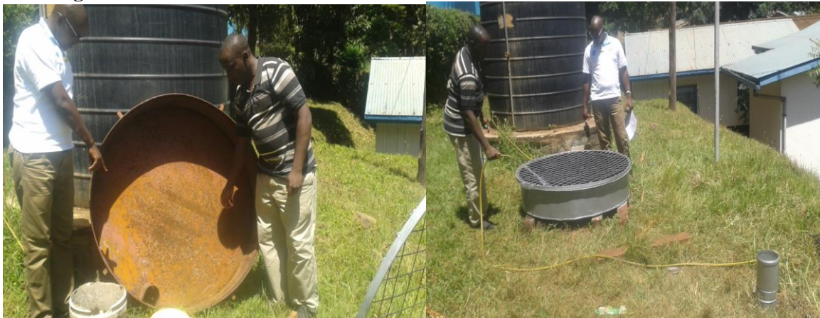
Removal of pan
