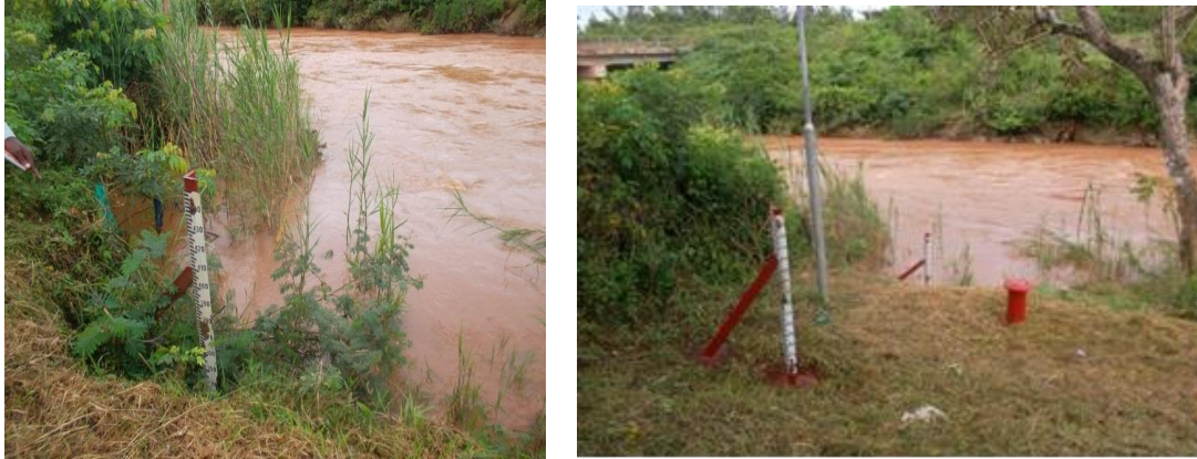
Figure 3.3: Rehabilitation works of Yala at Bondo Station (1FG02) in LVSCA
