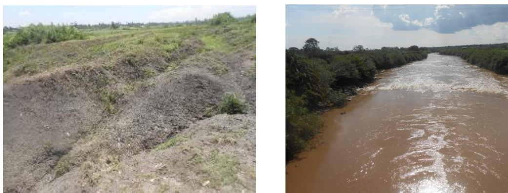
Figure 3.18: Gullies within Mid Nzoia (left) and Nzoia River downstream of Musanda Bridge (right)
