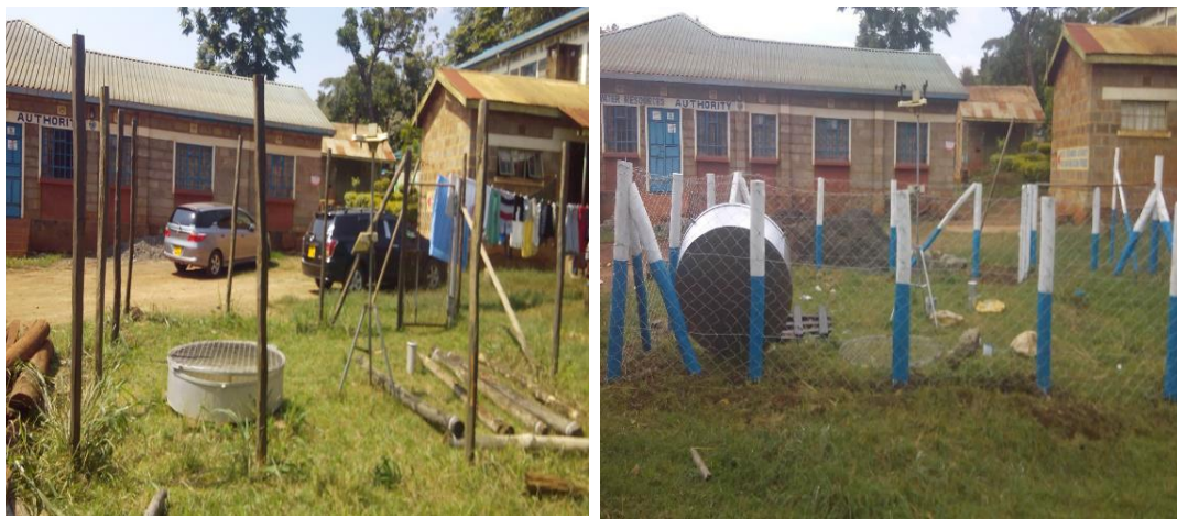
Figure 2.2: Murang'a Met station before and after installation
