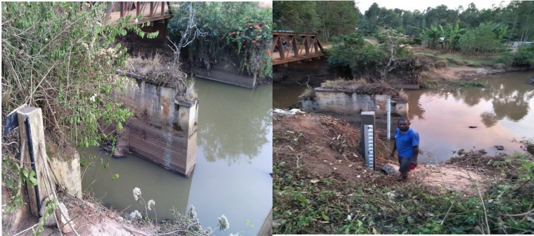
Figure 3.1:Yala-1FE02; Before (Erection of the pillar) and after (1st & 2nd gauges installed) the installation.
