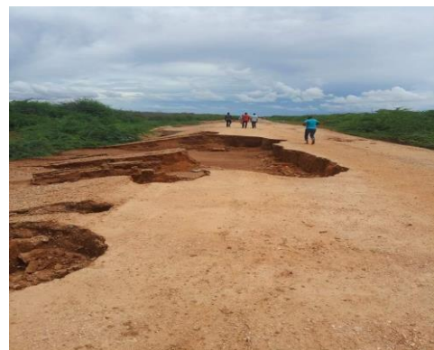
Road destruction in Garissa
