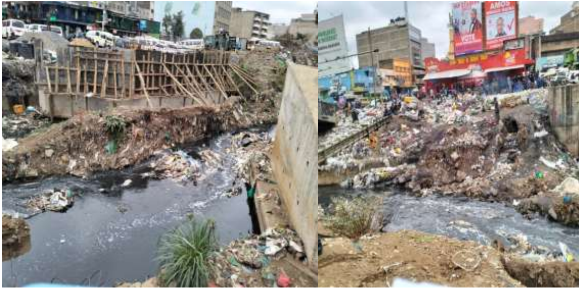
Figure 3.36 Unsorted Solid waste dumpsite -Racecourse Bridge
