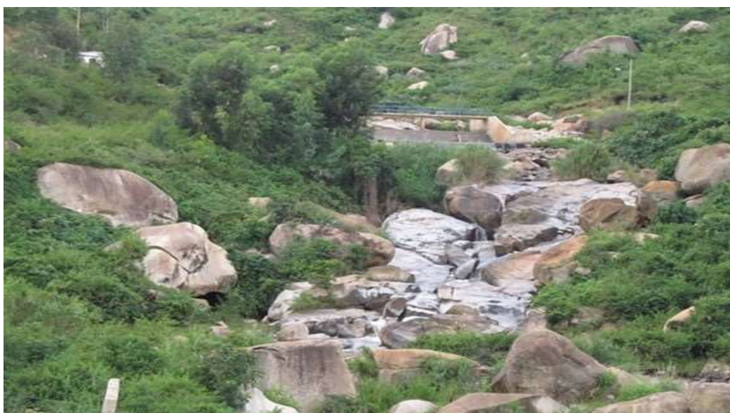
Figure 6-25: Diversion weir on Kajulu River
